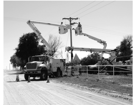
▲ Electric lineworkers perform a variety of tasks in their jobs, including working on overhead lines and substations.
